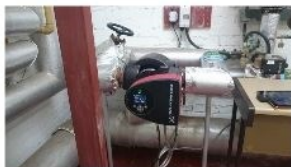
A recent installation with a Grundfos heating pump. This pump has been fitted with two temperature sensors to enable it to have a 10° differential set-point
